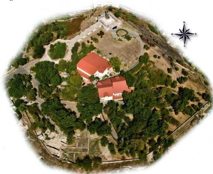
Fig. 2. Aerial photograph of the Monument Park (after Mocanu, Nuțu 2017)
