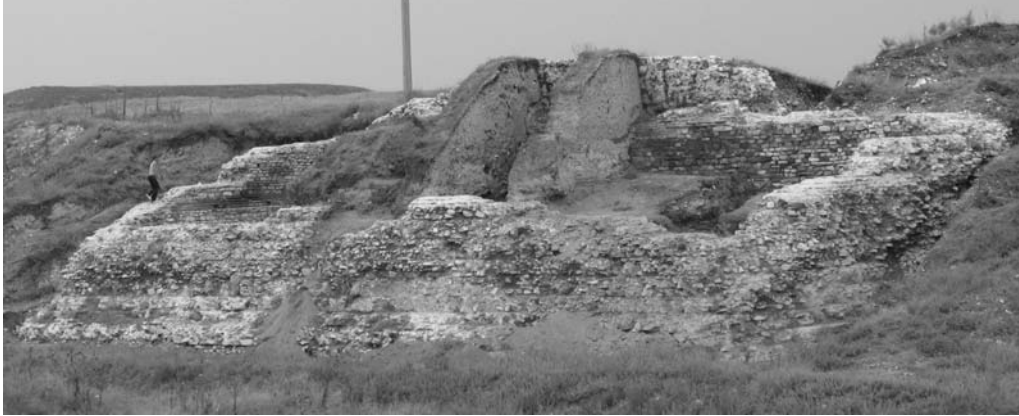
Figure 4. The large tower at Noviodunum in 2004.
